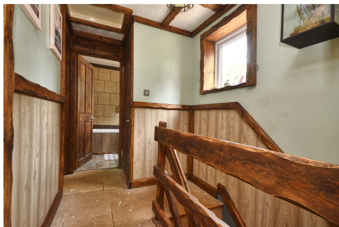
First Floor Landing
